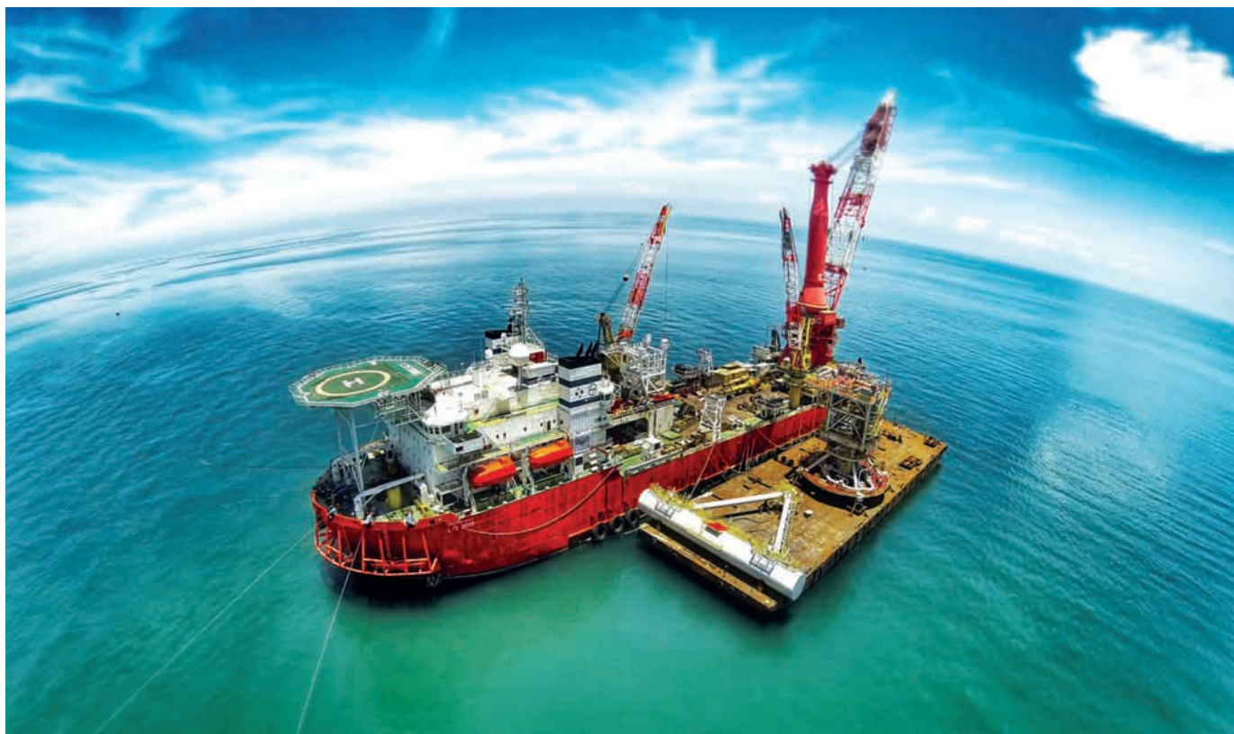
Tower Yoke Mooring facility installation by LTS3000 at Lampung field, Indonesia.
