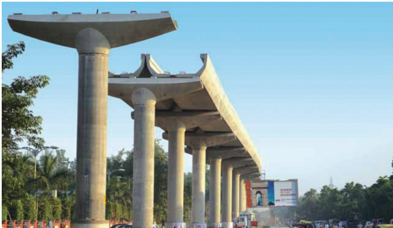
Viaduct under construction which uses the new precast technology: 'U' girder.
