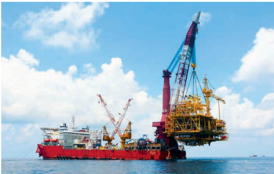
LTS3000 lifting 2719 MT CPP Topside.
